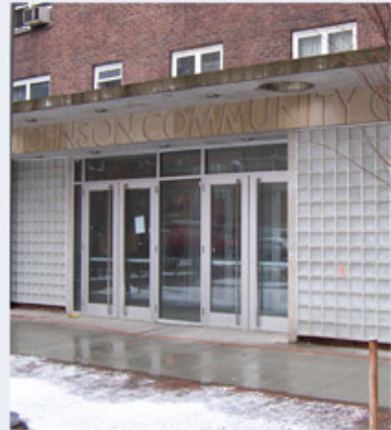
Johnson Community Center.
